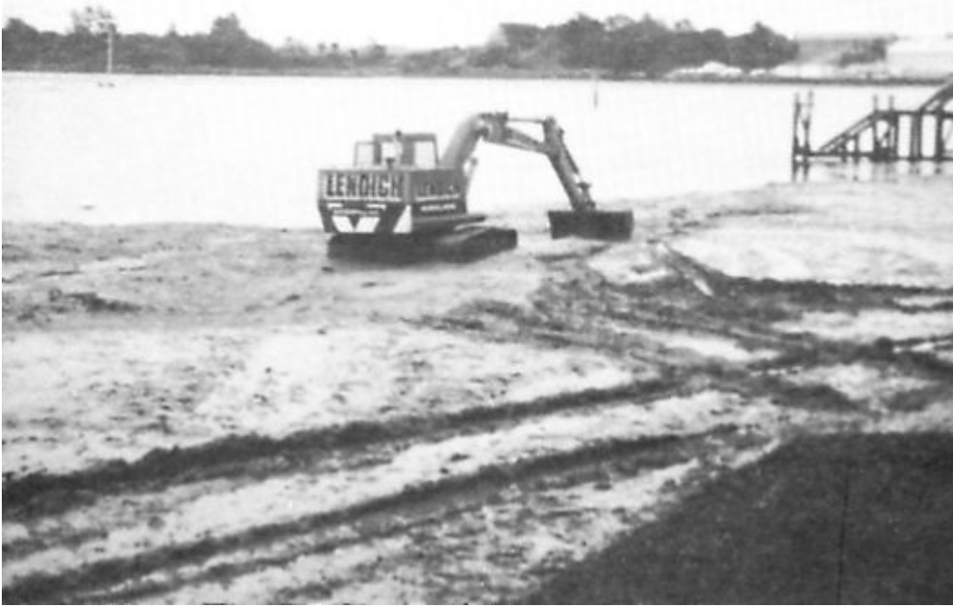
Final stage of clearing mud from the sea bed.
