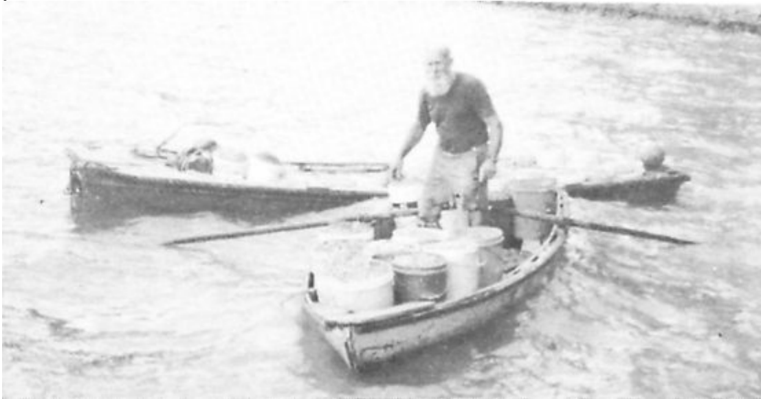
Unloading sand at full tide by the groyne.
