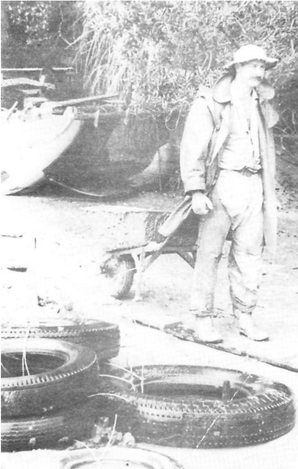
Ready to start 1st stage of the tyre groyne.
